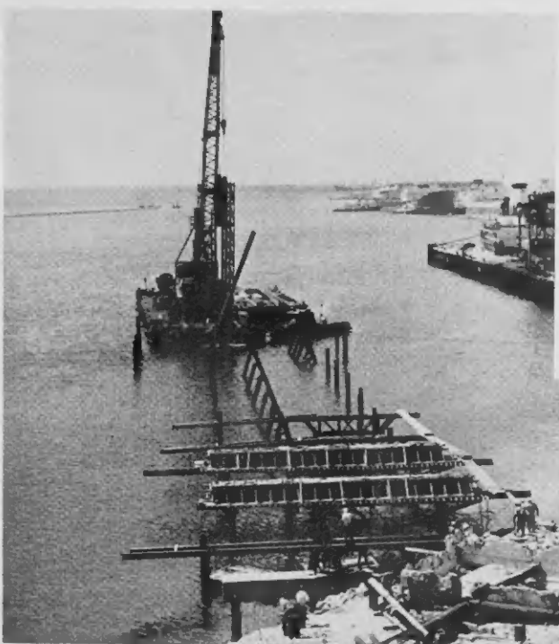
LAGO'S NO. 3 Finger Pier, above, begins to take shape as the first concrete caps on pilings are fitted. The area near the police station in Oranjestad, below, takes on a new look with new traffic islands. FINGER PIER No. 3 di Lago, ariba, ta cuminza haya forma cu sintamento di e promer cabezonnan di concreto bashá ariba e pilanan. E vecindario banda di warda di poliz na Oranjestad, abao, ta haya un aspecto nobo cu e islanan nobo di trafico.
